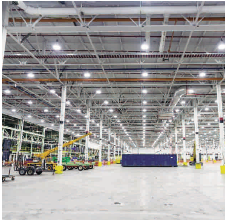
Former material consolidation area at the Marysville Auto Plant will create a new workspace where the IPU will be sub-assembled. (HONDA PHOTO)
